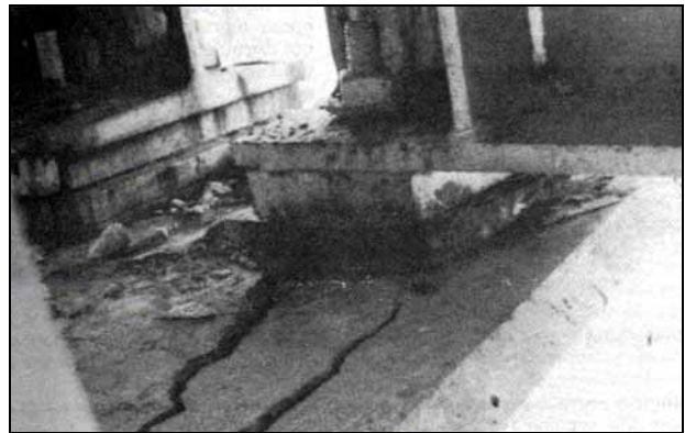
Exhibit X. 25 Crack in Seat
